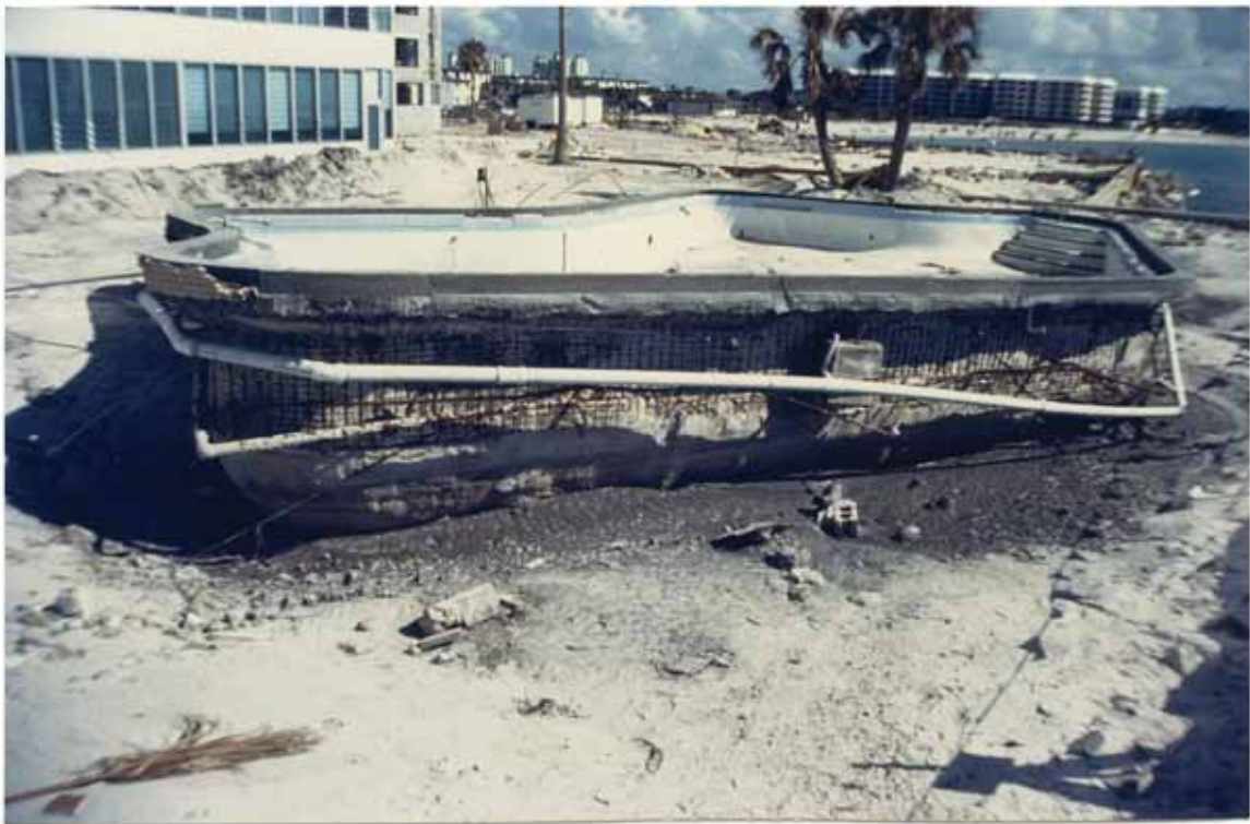
FIGURE 124. Pool at Starlight Tower Condominium floated above grade during Juan's flooding, St. Petersburg Beach
