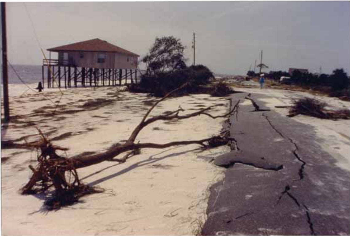
FIGURE 33. Elena erosion and damage
