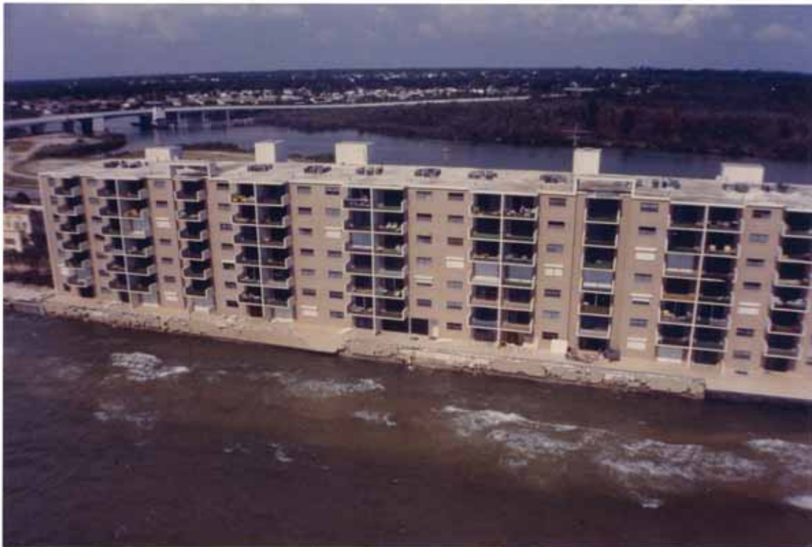
FIGURE 114. Gulf Shores Condominium after Elena
