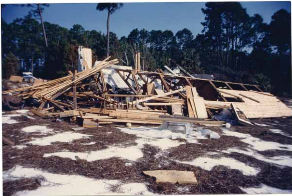
FIGURE 21. Carrabelle Beach dwelling destroyed by Elena
