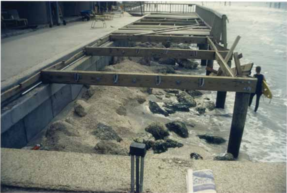
FIGURE 100. Toe-scour protection after Juan
