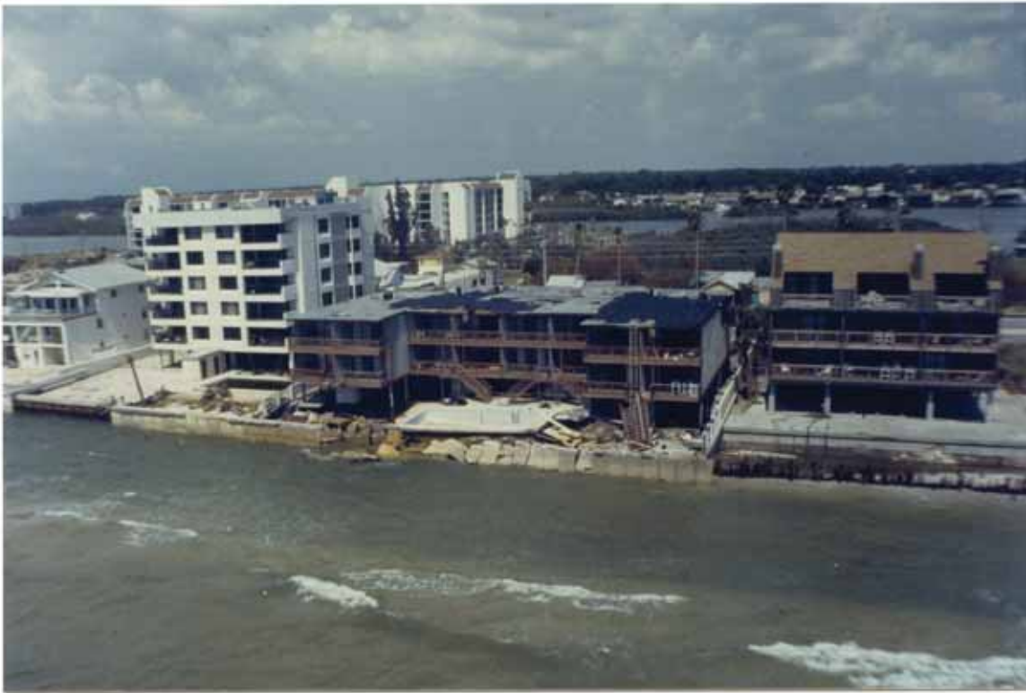
FIGURE 113. Bulkhead destroyed by Elena
