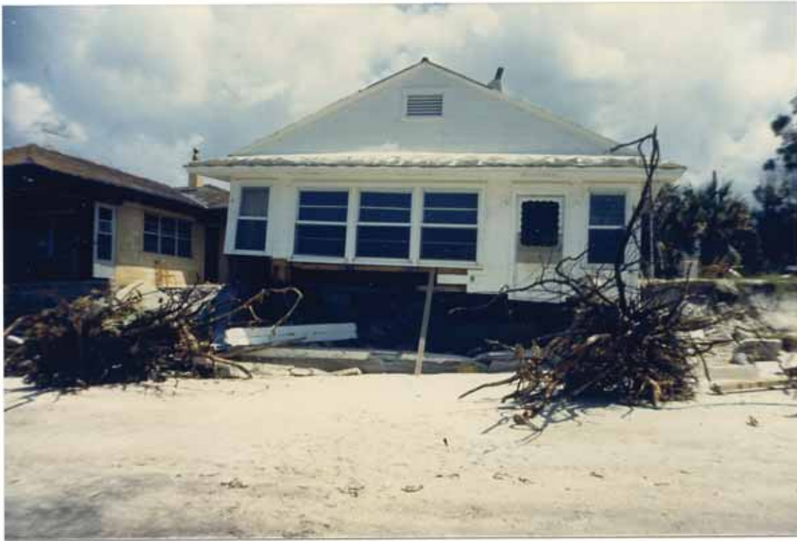
FIGURE 86. Dwelling damaged by Elena
