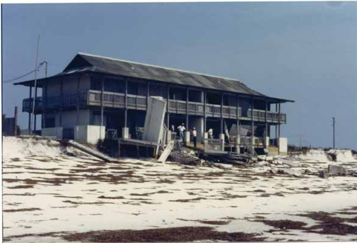
FIGURE 13. Pelican Inn damaged by Elena, Dog Island (G. L. Hill)
