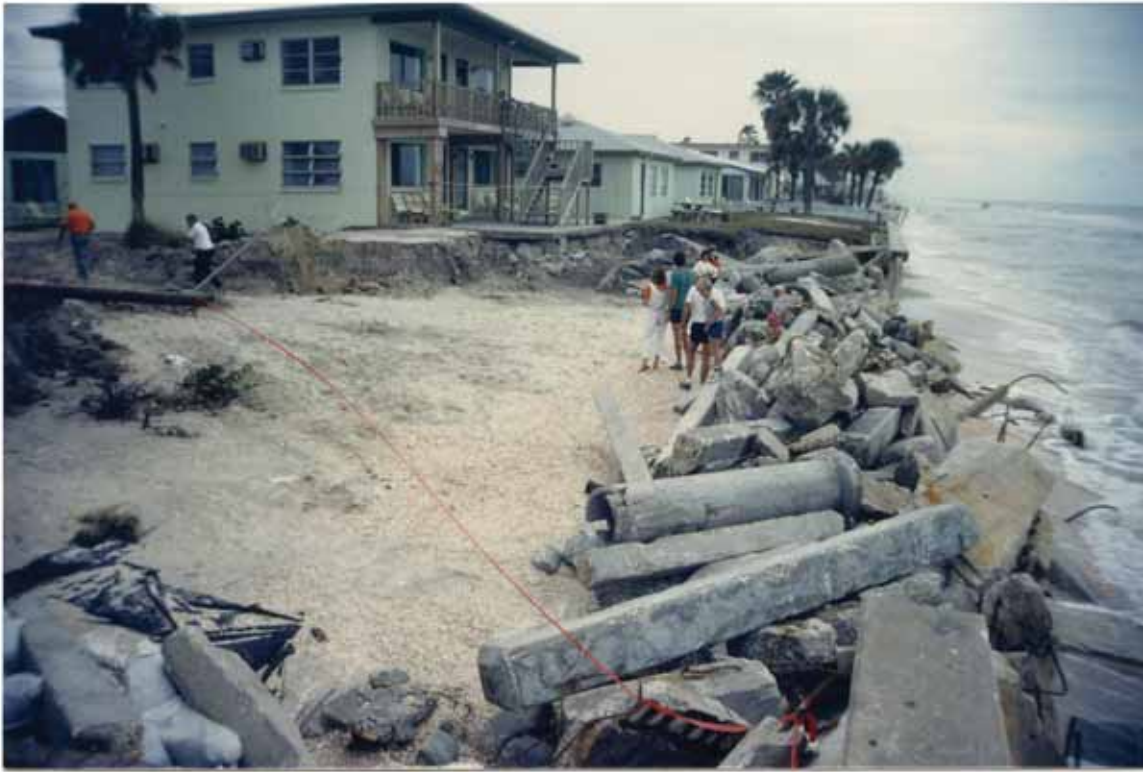
FIGURE 76. Juan destroyed 23rd Avenue
