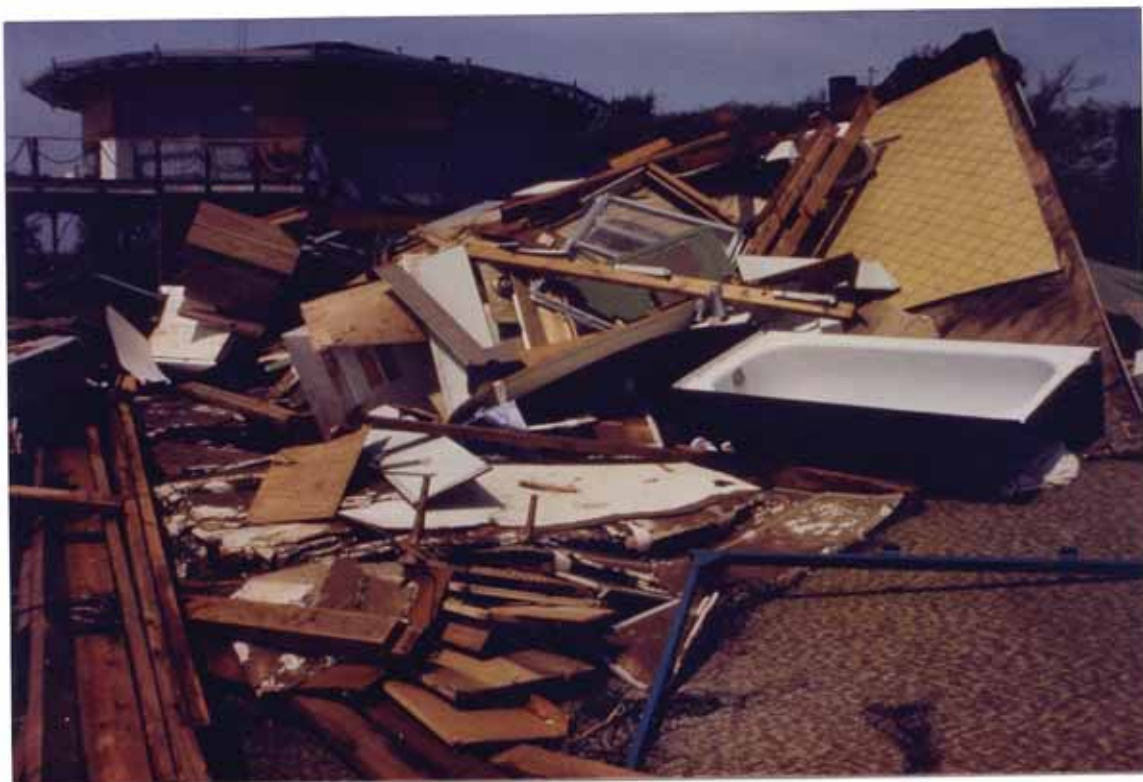
FIGURE 27. Southwest Cape dwelling destroyed by Elena
