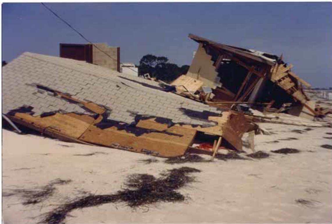
FIGURE 35. Same dwelling destroyed by Elena's erosion and waves on September 1
