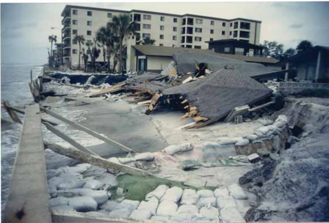
FIGURE 73. Same dwelling destroyed by Juan
