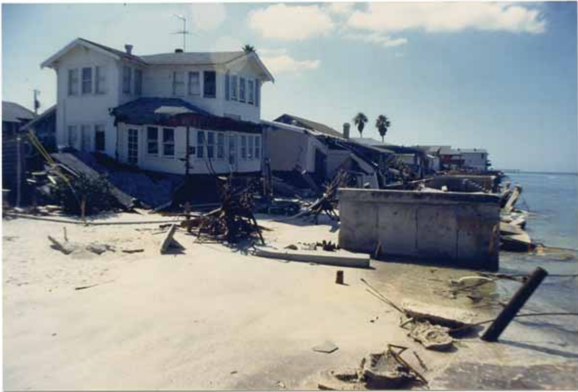
FIGURE 92. Elena destroyed 8th Avenue
