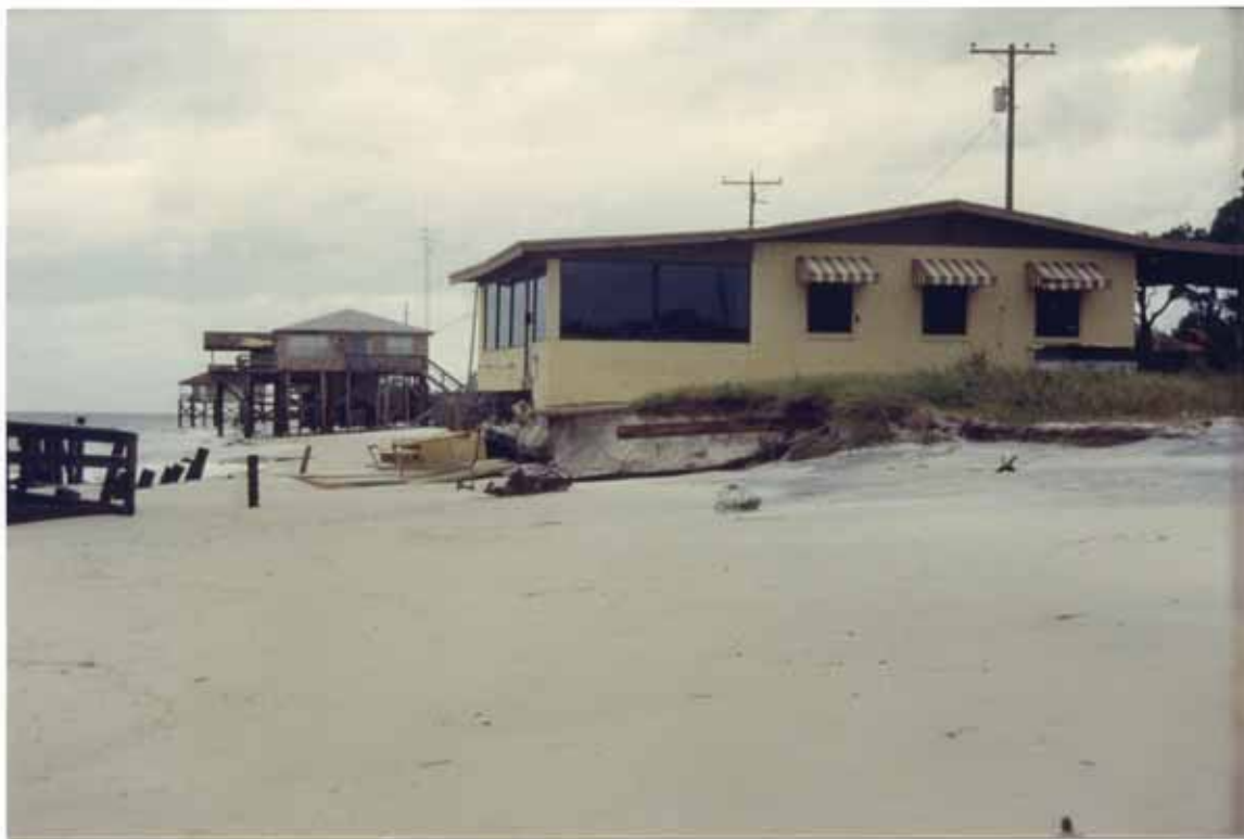
FIGURE 34. Wood bulkhead destroyed and dwelling undermined on August 30 (H. N. Bean)
