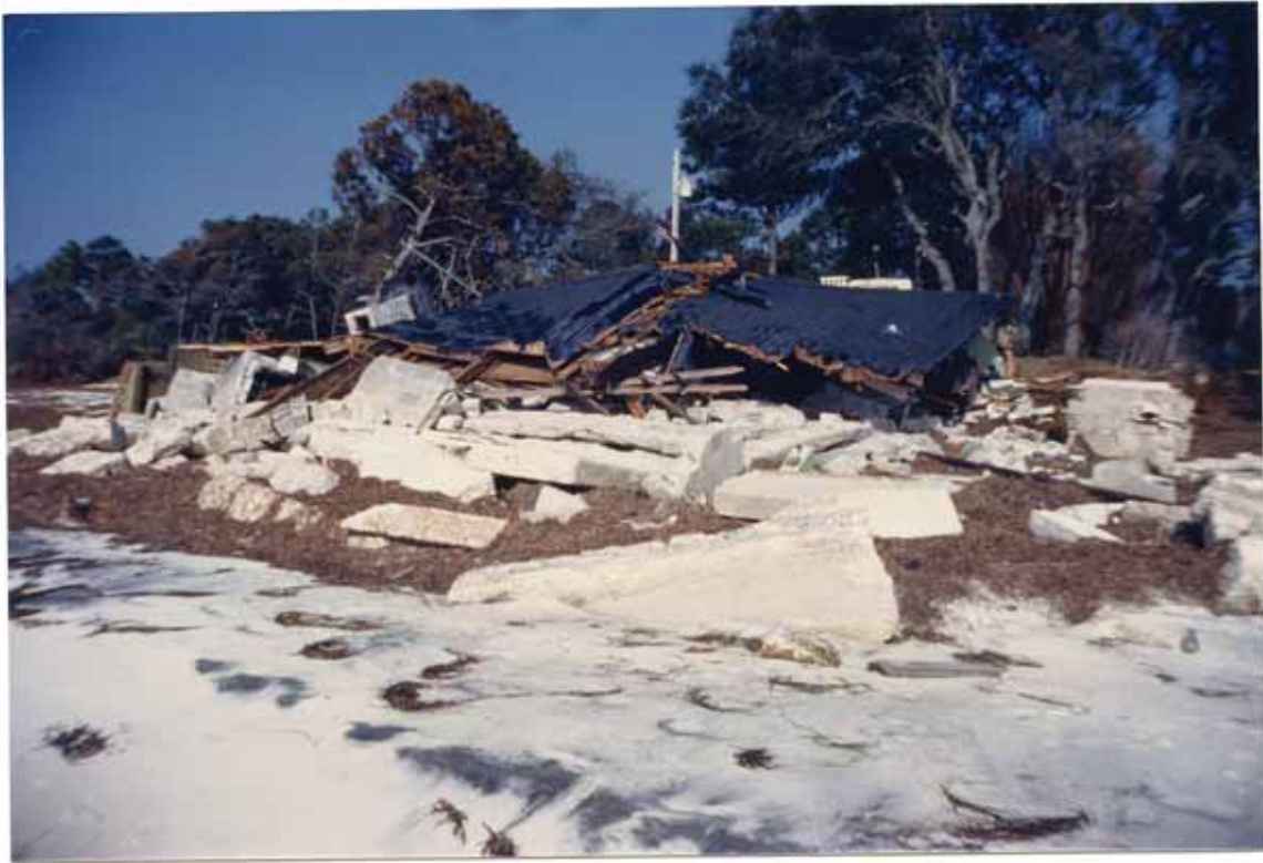
FIGURE 20. Carrabelle Beach dwelling destroyed by Elena
