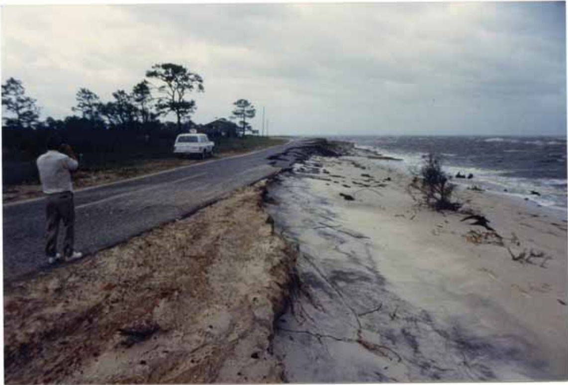
FIGURE 44. Lighthouse Point road damaged on August 30
