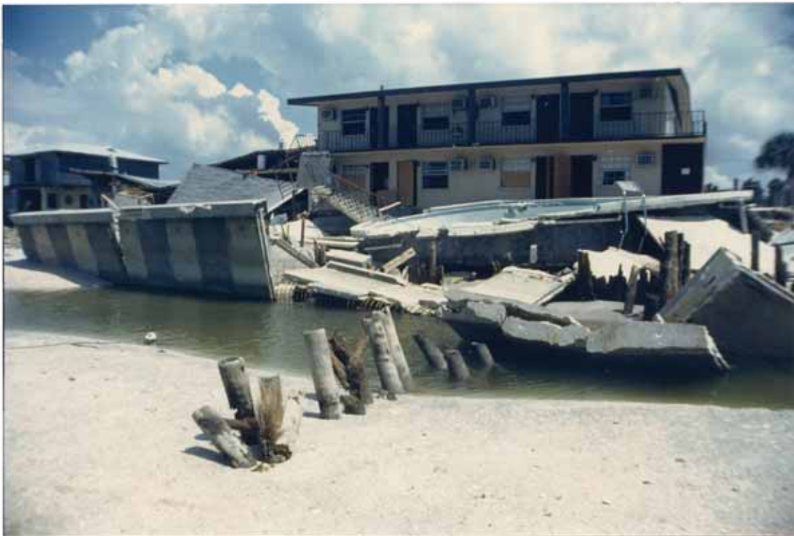
FIGURE 57. Bulkhead and swimming pool destroyed Chateau Motel, Belleair Beach
