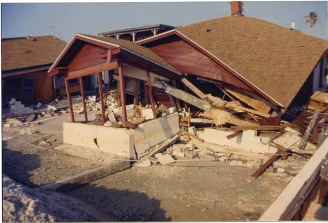
FIGURE 105. Dwelling destroyed by Elena
