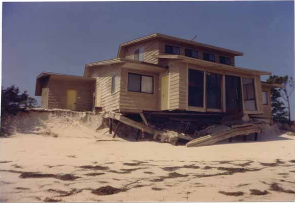
FIGURE 42. Lighthouse Point dwelling damaged by Elena's erosion
