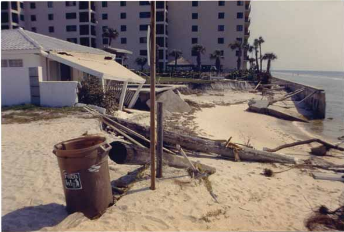
FIGURE 70. Damage at 25th Avenue, Indian Rocks Beach
