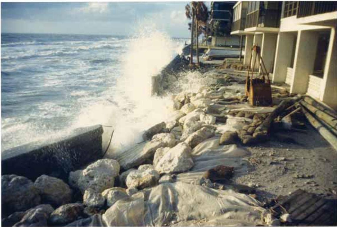
FIGURE 116. Emergency revetment protection from Juan
