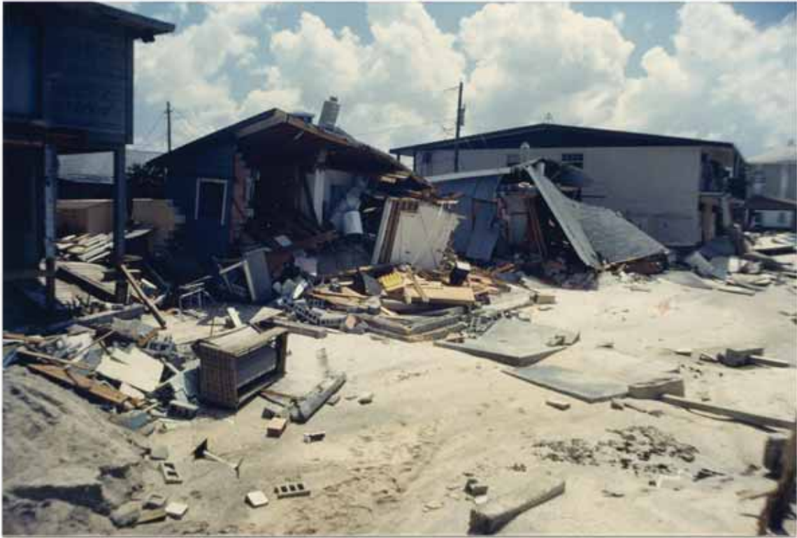
FIGURE 56. Belleair Beach dwellings destroyed by Elena
