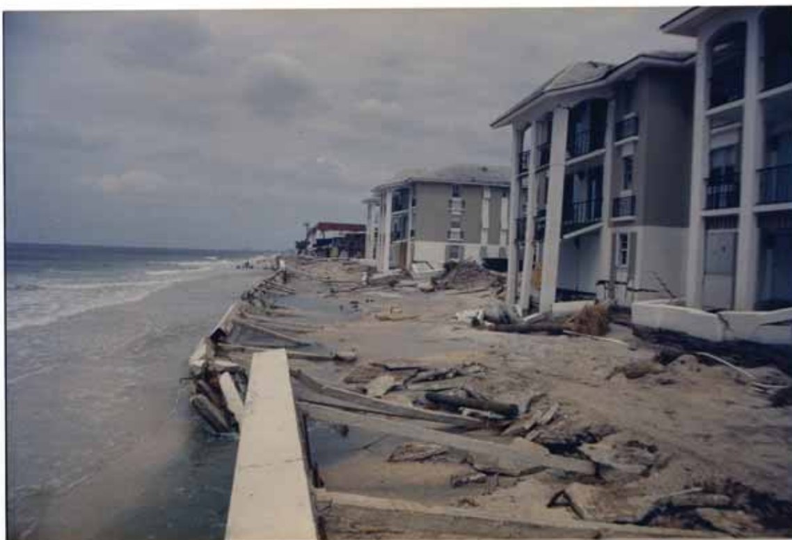
FIGURE 58. Tortugas Condominium bulkhead destroyed and buildings damaged
