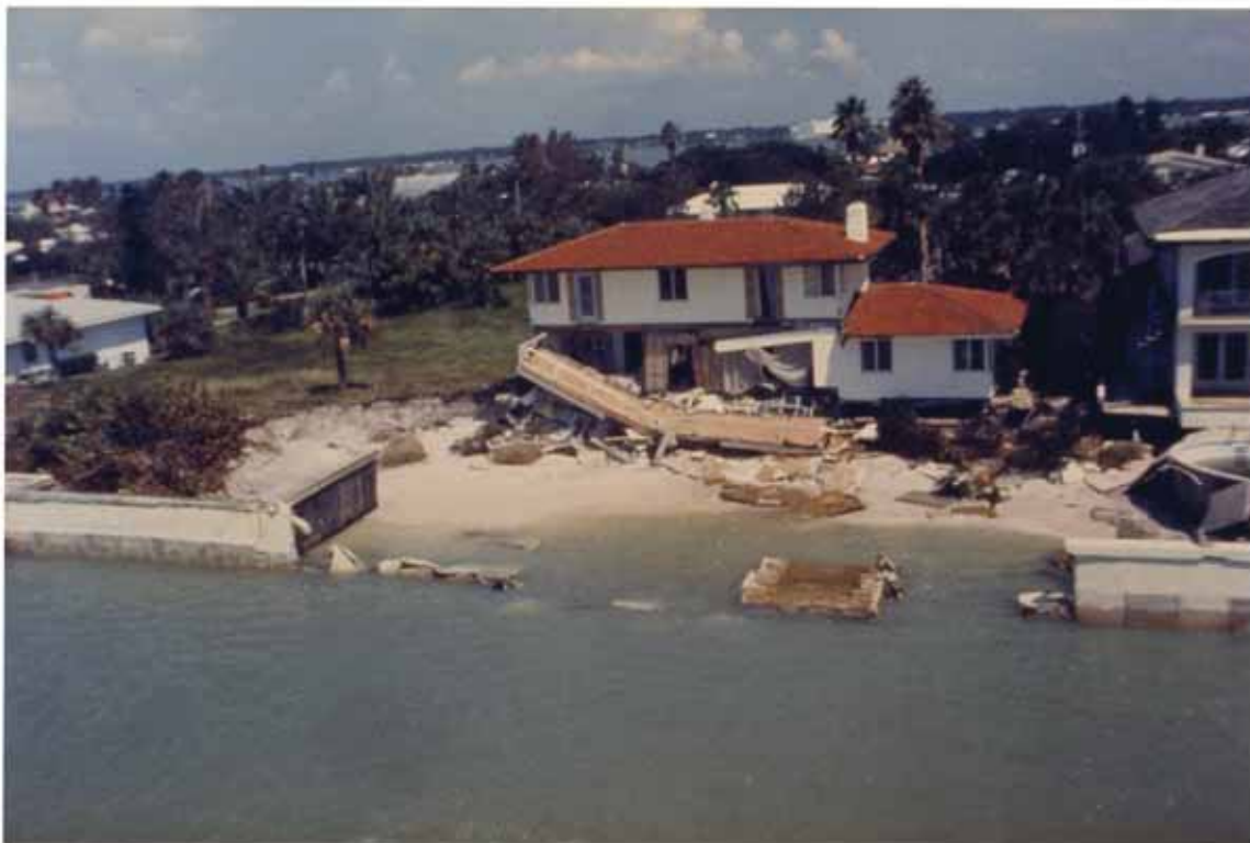
FIGURE 67. Wall destroyed and dwelling damaged
