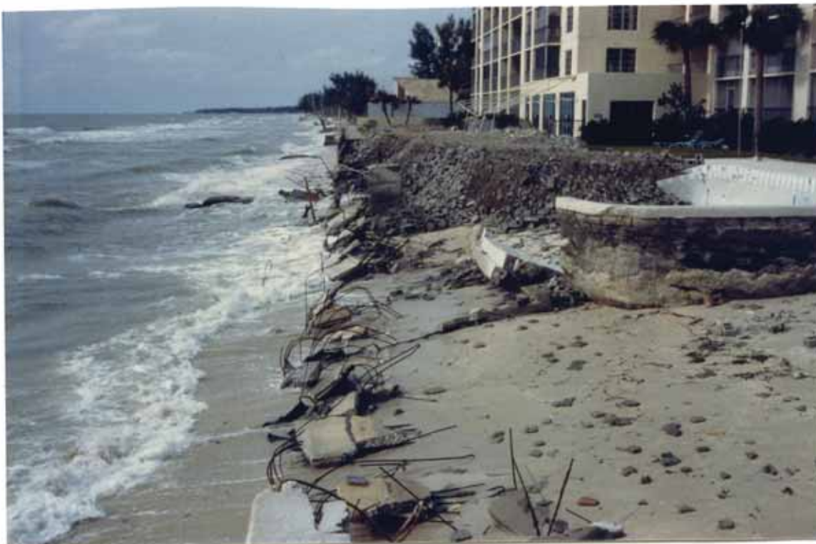
FIGURE 148. Juan destroyed pool and bulkhead, Longboat Harbor Towers (S. West)
