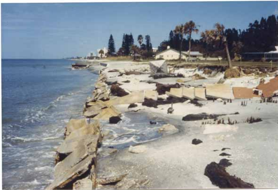
FIGURE 154. Elena destroyed Venice bulkhead (S. West)
