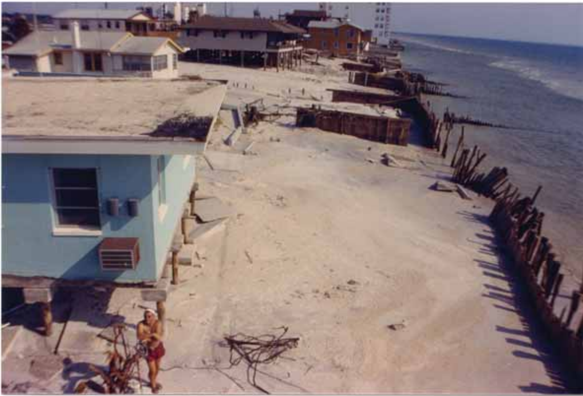
FIGURE 109. Indian Shores bulkheads destroyed, 820 feet
