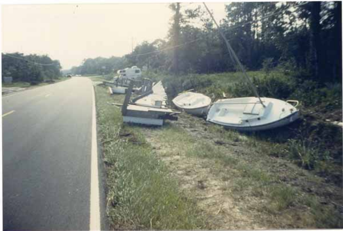
FIGURE 23. Elena's flooding at Lanark Marina, U.S. 98
