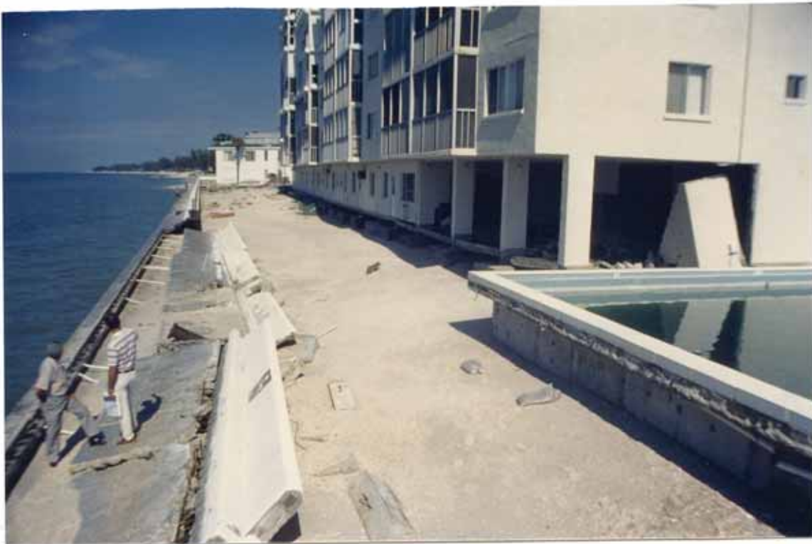
FIGURE 126. Juan destroyed sloping wall at Martinique Condominium
