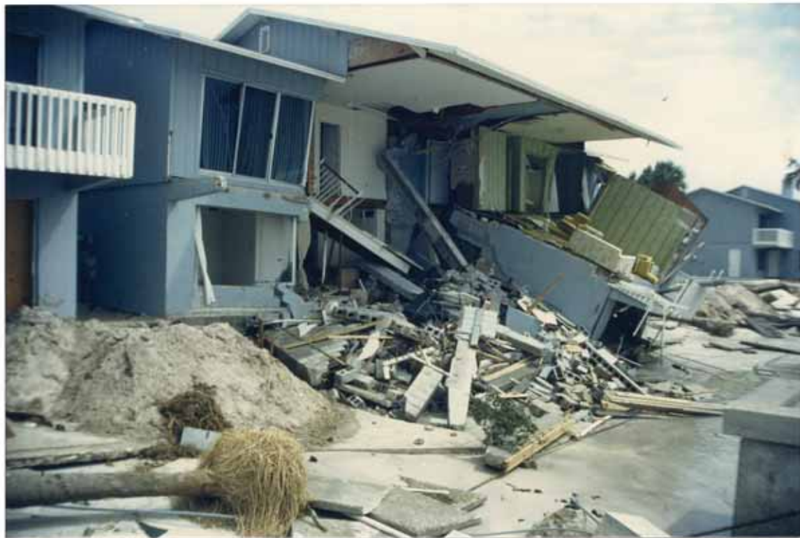
FIGURE 61. Two-unit building destroyed by Elena's waves
