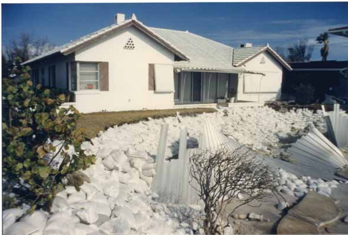
FIGURE 118. Emergency protection after Juan
