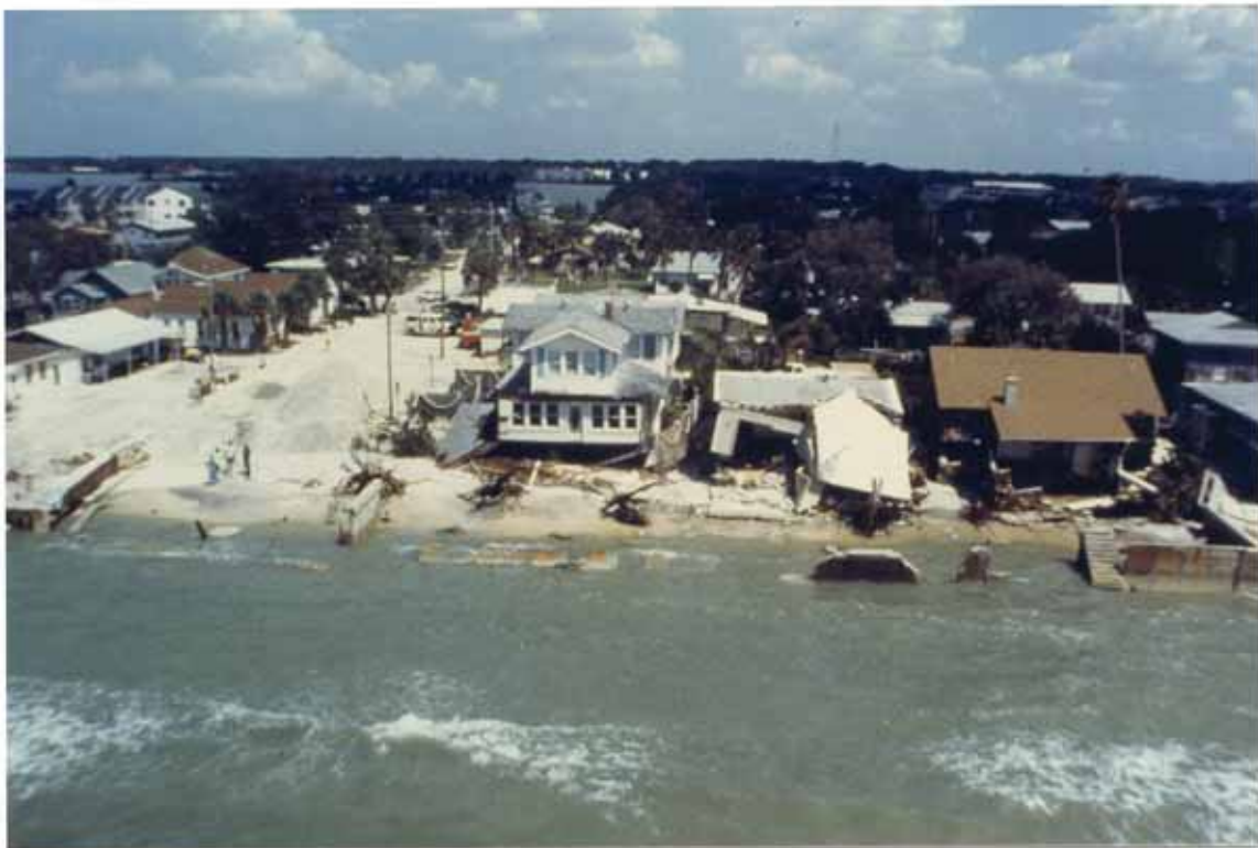
FIGURE 91. Bulkheads and dwellings destroyed and damaged
