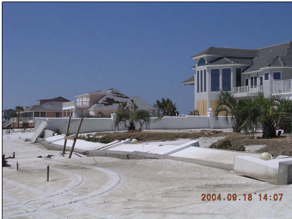
Photo OK-7. Overwash and decorative wall damage near R22 in Destin.
