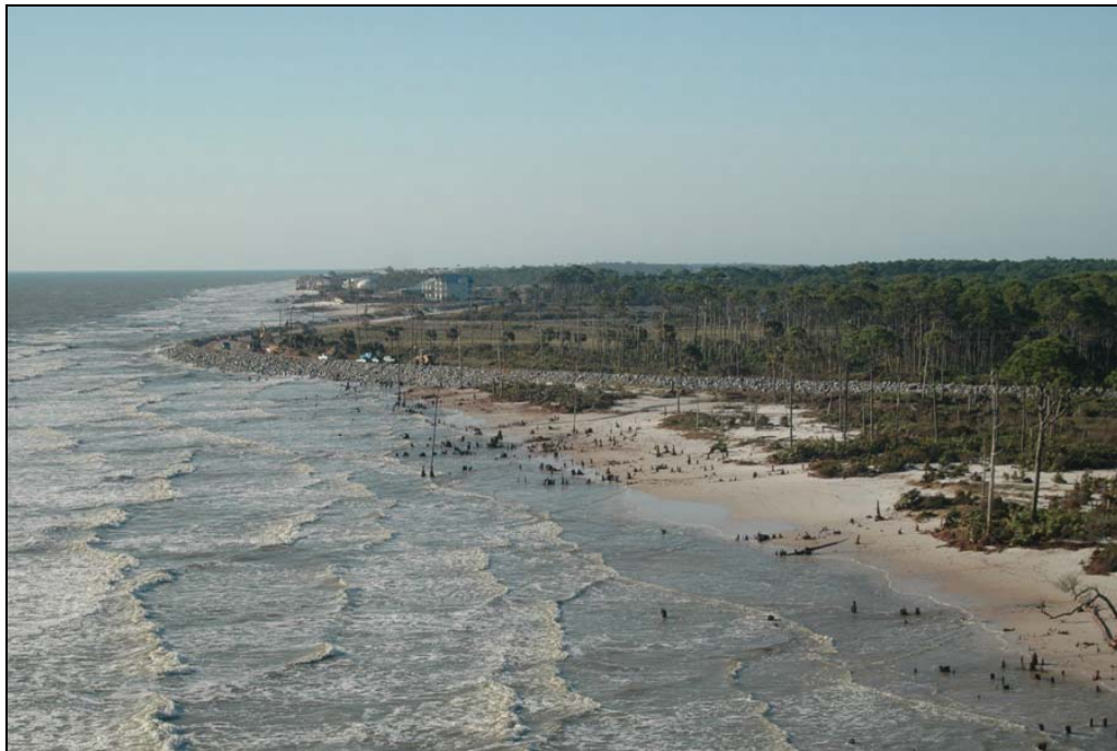
Photo GU-8. Revetted County Road 30E at "Stump Hole" on St. Joseph Peninsula at R105. (Note: The road was substantially seaward of the shoreline prior to Ivan).
