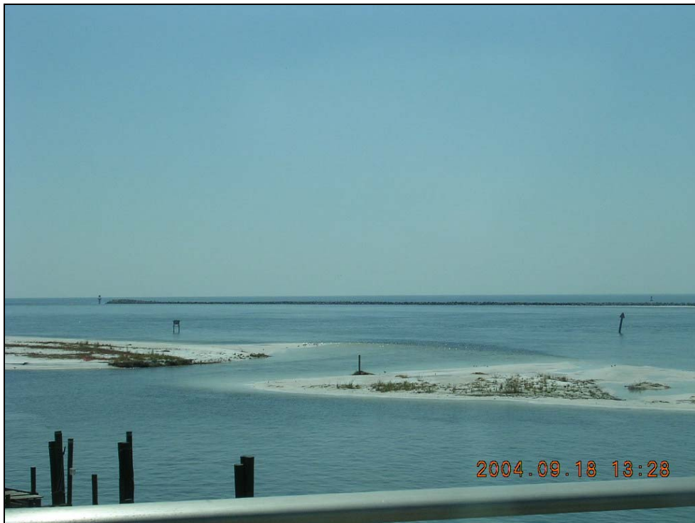
Photo OK-6. Breach through Norriego Point at Destin-East Pass.
