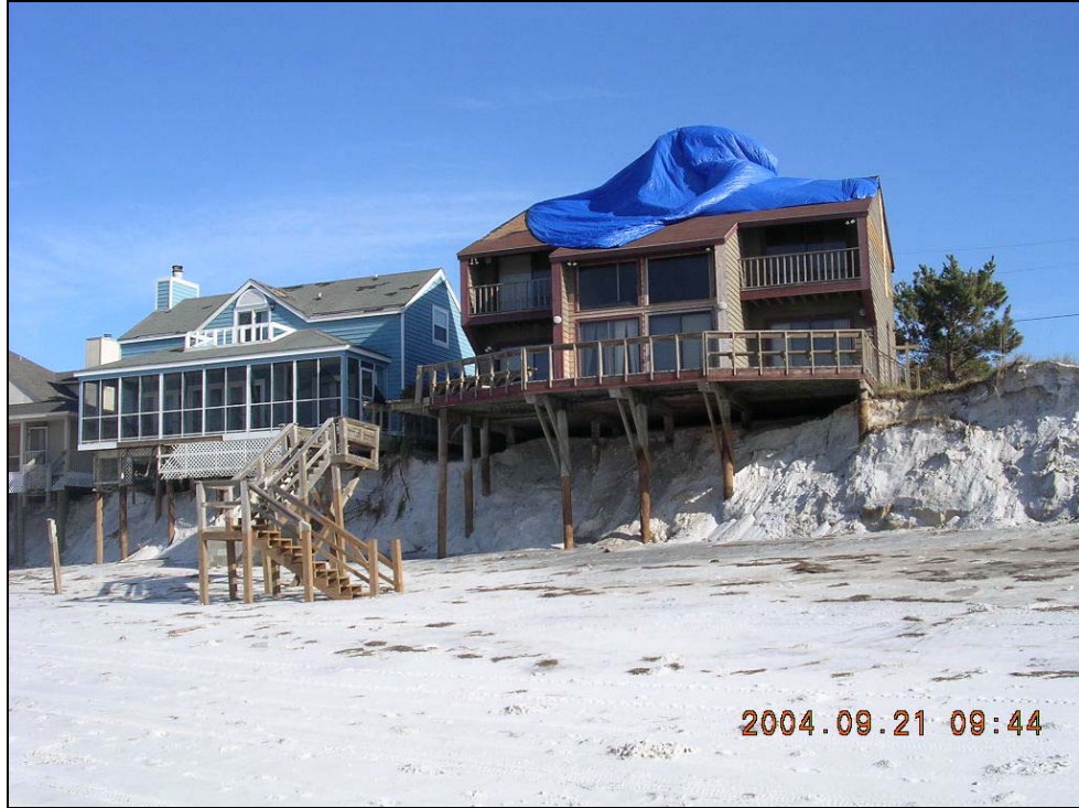
Figure WL-10. Eroded dune undermining houses at R123 at Inlet Beach.
