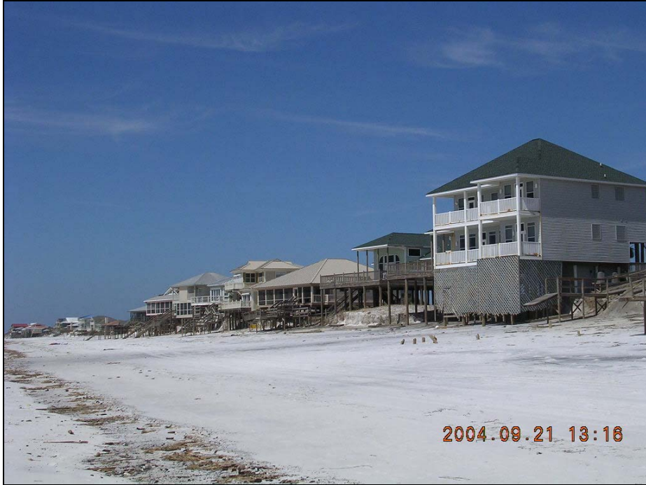
Photo WL-6. Habitable structures in relation to beach and dune at R47 (+250') in the Beach Highlands/Dune Allen area.
