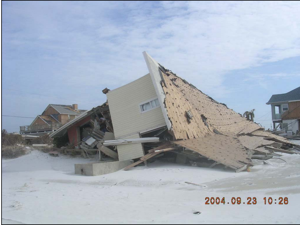
Photo ES-14. Destroyed single-family dwelling at R126 (+100') in Pensacola Beach.
