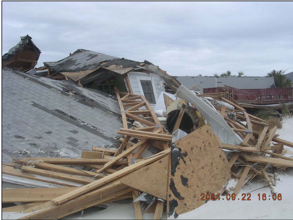
Photo ES-18. Destroyed single-family dwelling at R137 (+50') in Pensacola Beach.
