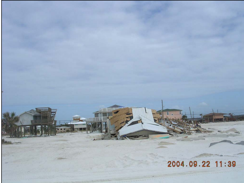
Photo SR-3. Destroyed single-family dwelling at R204 (+500') in Navarre Beach.
