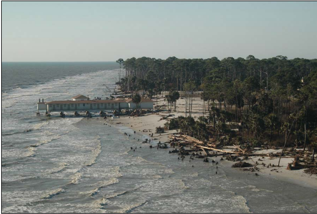
Photo GU-9. Old Coast Guard barracks after Ivan at R110 (-250') (Note: the building was located substantially seaward of the shoreline into the Gulf waters prior to Ivan).
