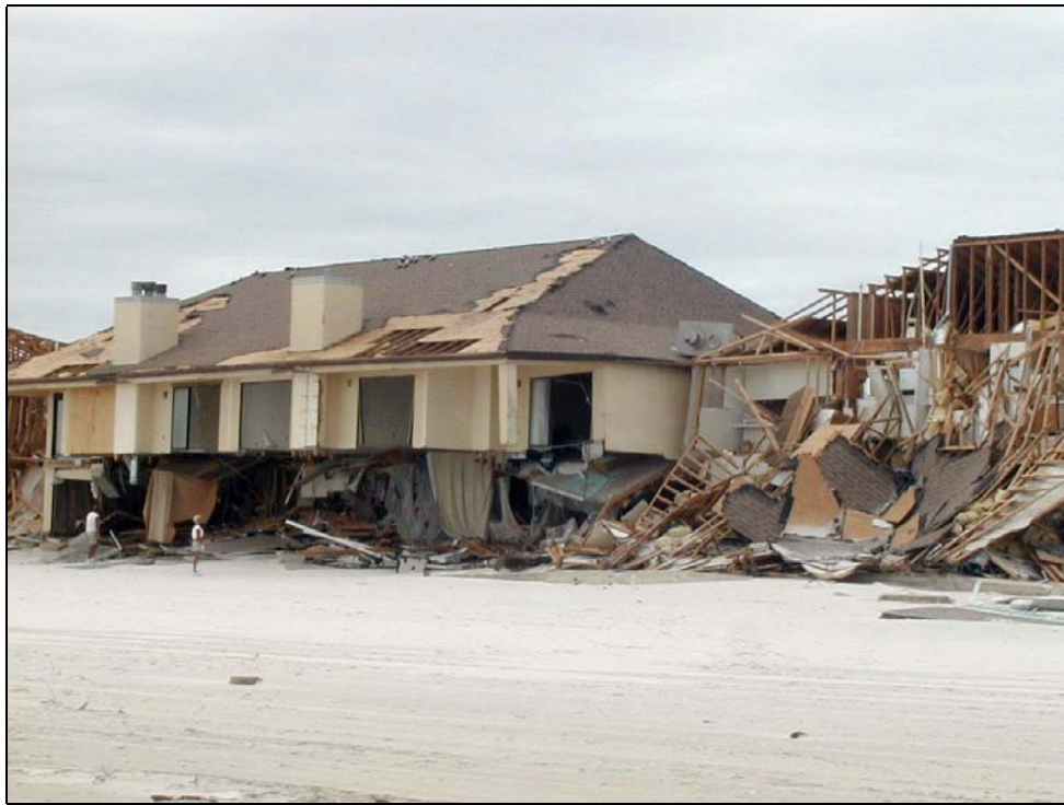
Photo ES-4. Destroyed single-family dwellings at R27 in Perdido Key.
