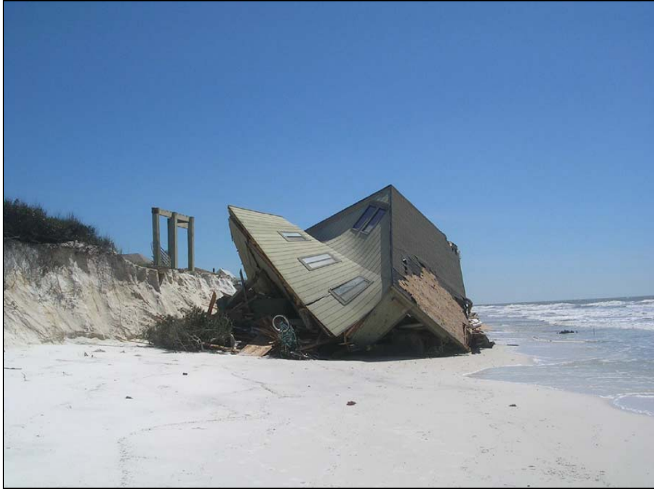
Photo GU-3. Destroyed single-family dwelling on St. Joseph Peninsula at R101 (-400')
