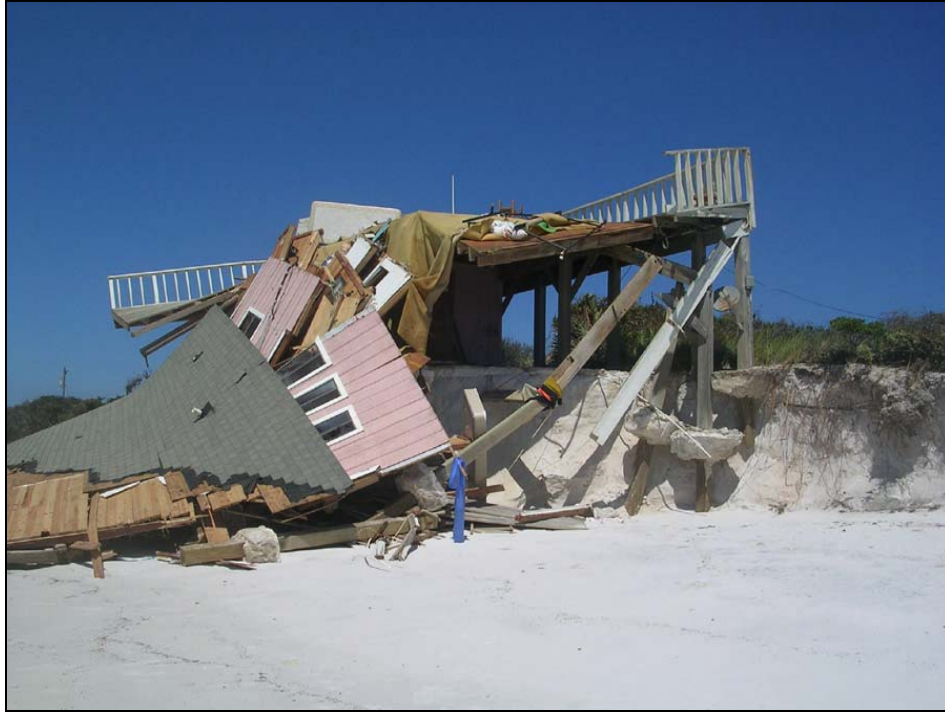
Photo GU-1. Destroyed single-family dwelling on St. Joseph Peninsula at R100 (+450')
