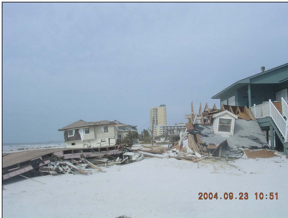
Photo ES-13. Destroyed single-family dwelling at R125 (+500') in Pensacola Beach.
