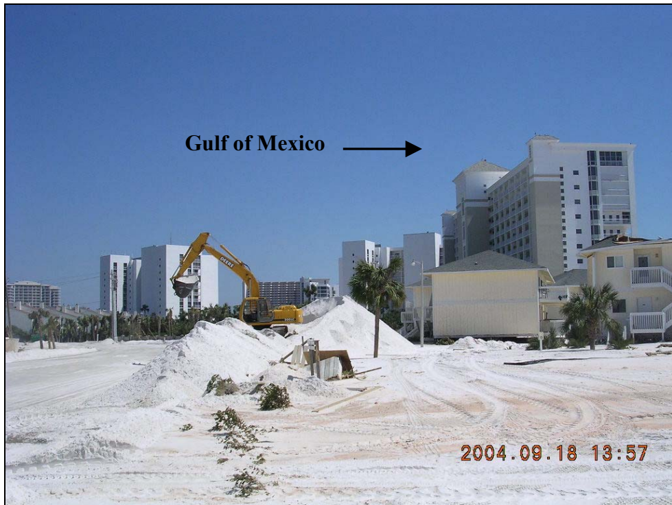
Photo OK-8. Extensive overflow of beach sand and road clearing in Destin at R24-25.
