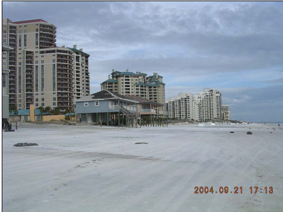
Photo WL-4. Structures located on or very near the beach at R18 (+200').
