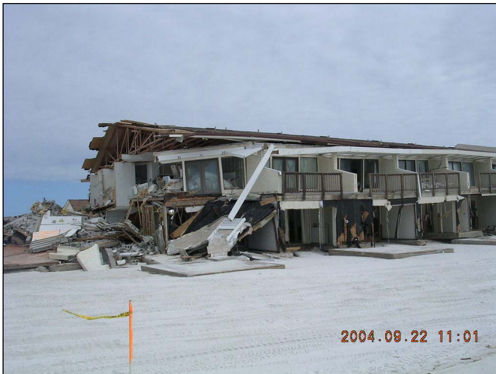
Photo SR-4. Destroyed multi-family dwelling structure at R208 (-200') in Navarre Beach.
