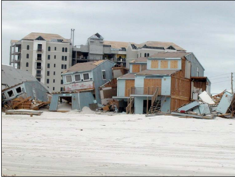
Photo ES-3. Destroyed multi-family dwellings at R22 (+450') on Perdido Key.
