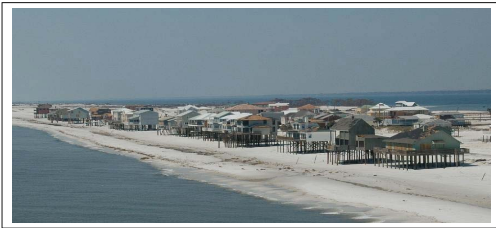
Major beach erosion at habitable structures City of Navarre Beach
