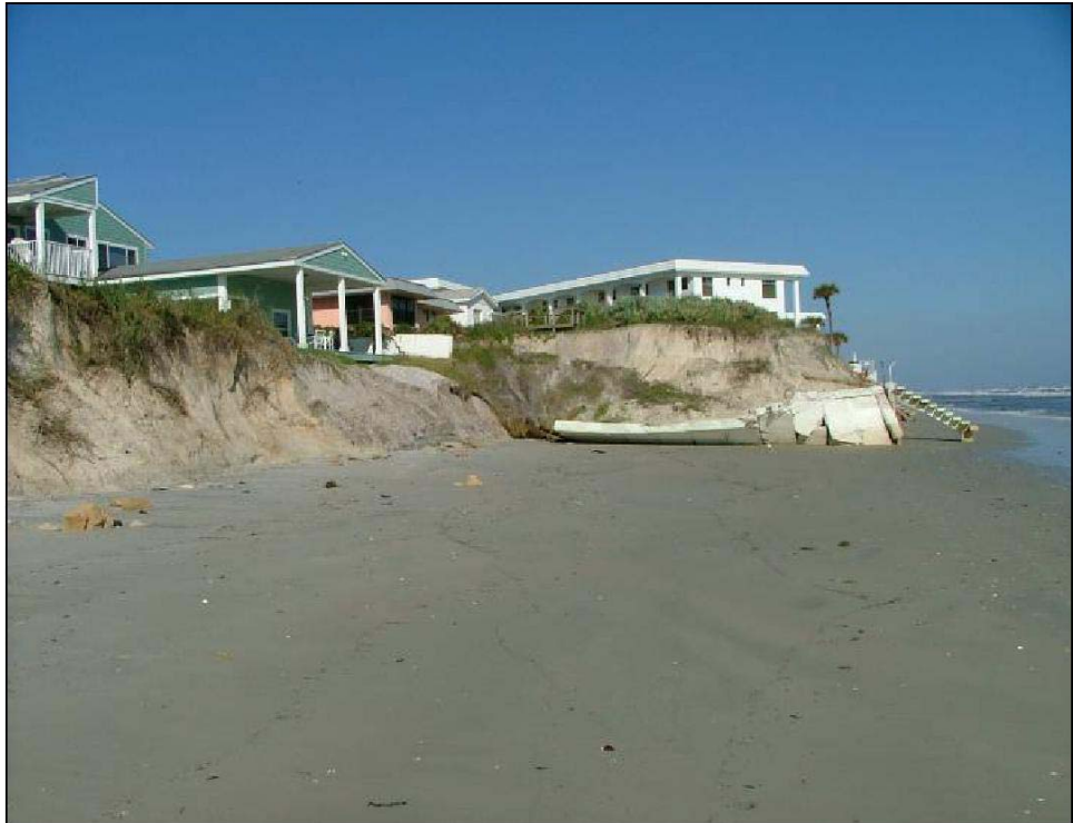
Photo 86. Wall destroyed and dwelling threatened, New Smyrna Beach (R167.1).
