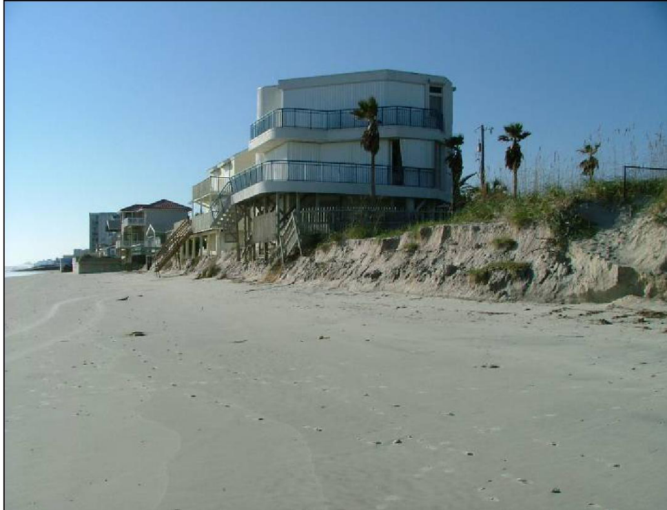
Photo 77. Threatened single-family dwellings along North Atlantic Avenue (R161).
