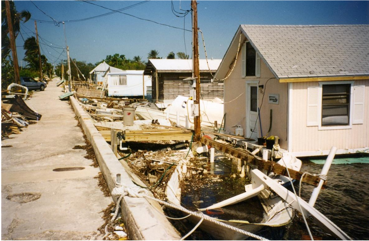
Damage along South Roosevelt Boulevard, Key West.
