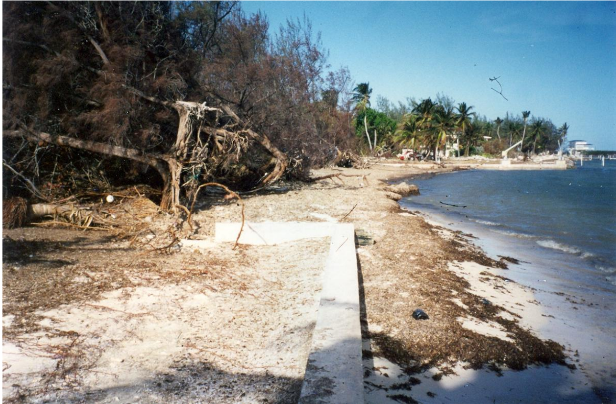
Damage at Lower Matecumbe Key.
