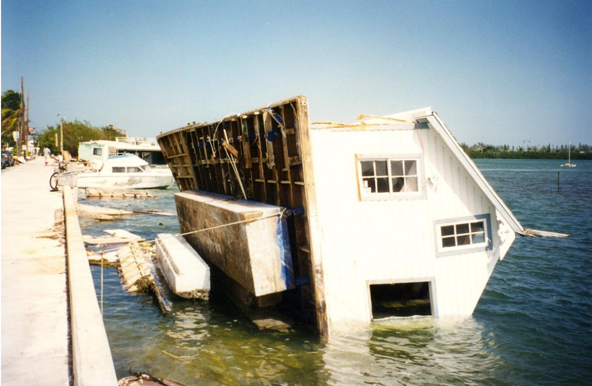
Damage along South Roosevelt Boulevard, Key West.
