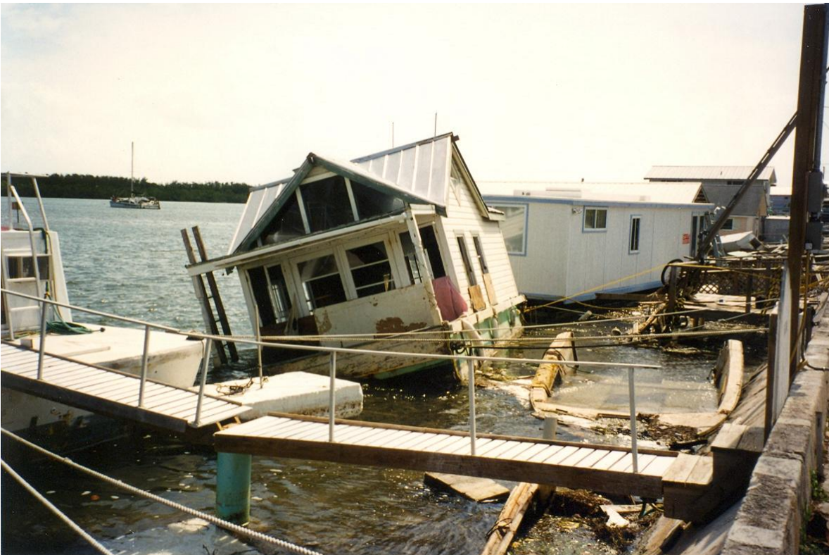
Damage along South Roosevelt Boulevard, Key West.
