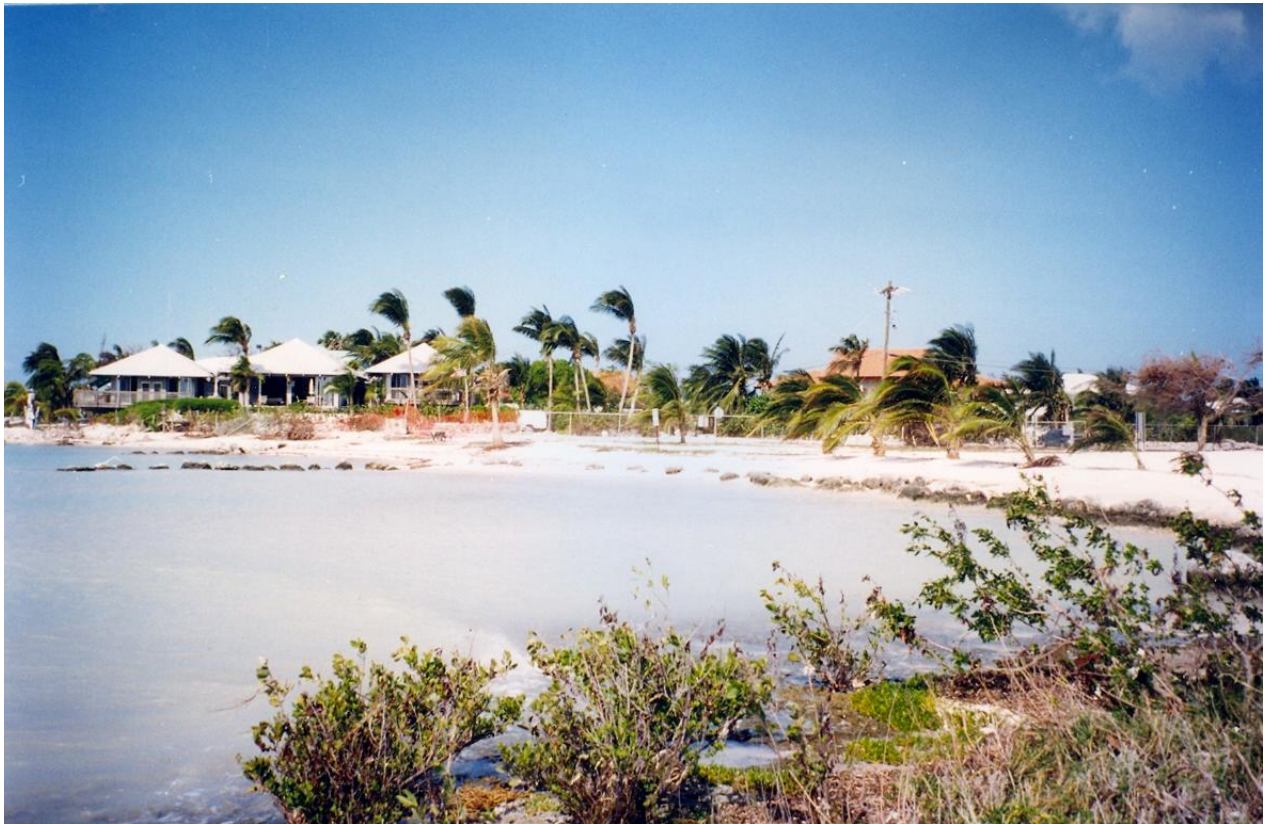
Damage at Sombrero Beach.
