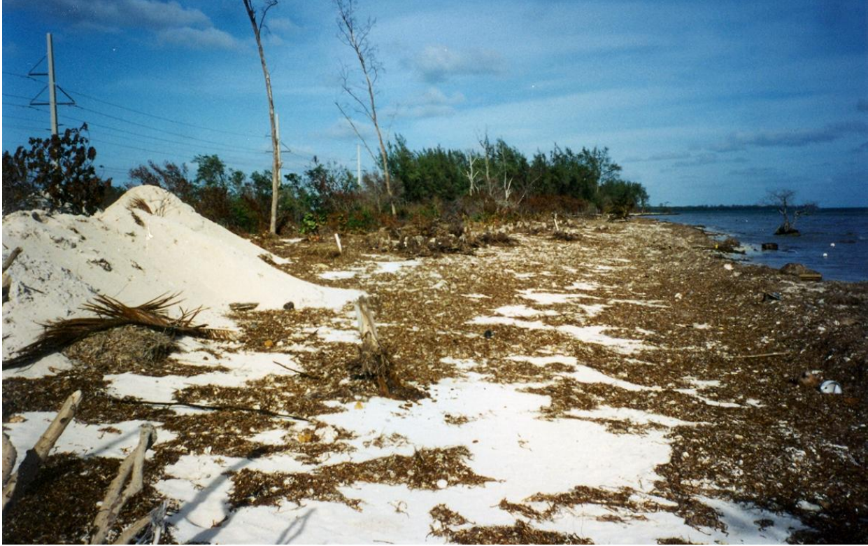
Damage at Long Key.
