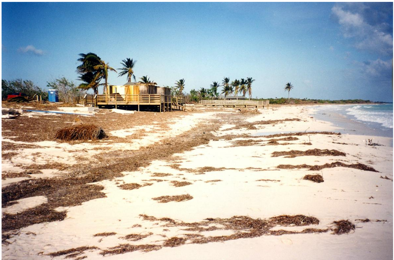
Conditions and damage at Sandspur Beach.
