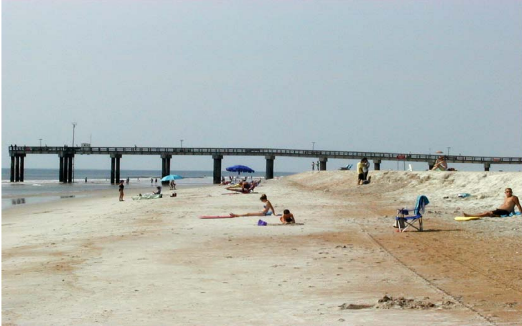
Photo 3. St. Augustine Beach Fishing Pier substantially landlocked following the federal beach restoration project [BBCS Photo Files]
