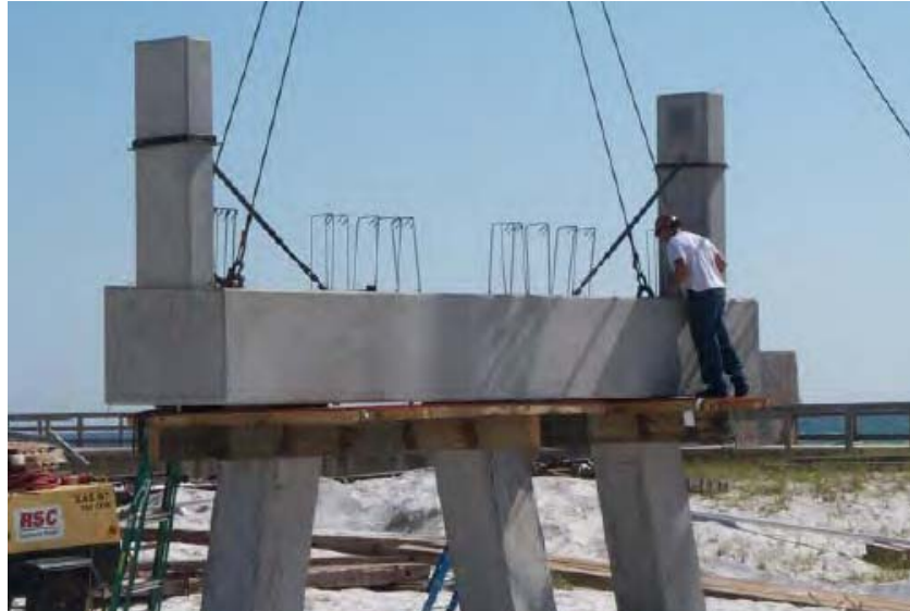
Photo 47. Cap placement on piles to construct pile bent [PBS&J]
