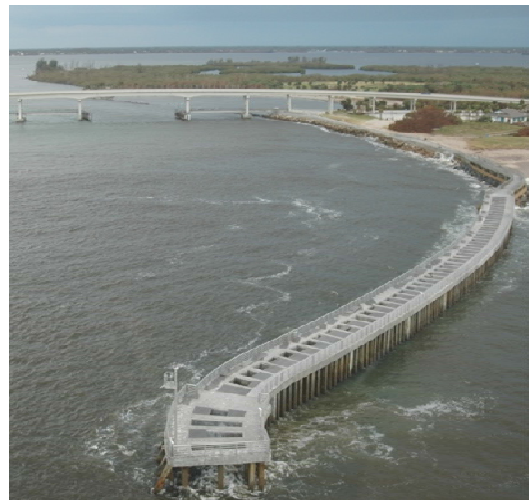
Photo 28. Pensacola Beach Fishing Pier before and after Hurricane Dennis’ wave uplift forces dislodged breakaway deck panels and rails without structural damage to the pier [BBCS Photo Files]
