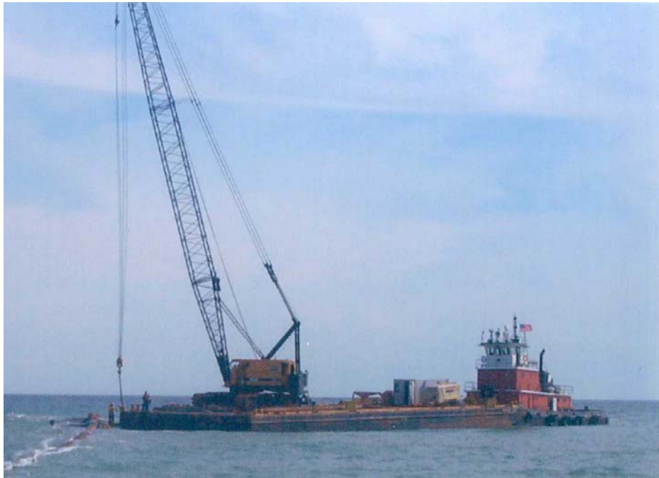
Photo 34. Barge and construction crane [BBCS Photo Files]
