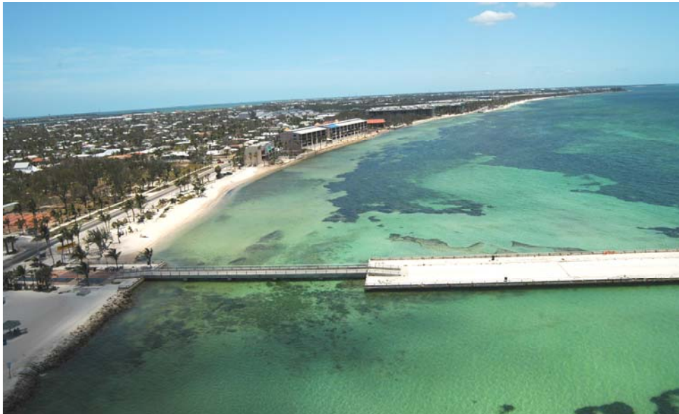
Photo 56. White Street Pier, Key West [BBCS Photo Files]
