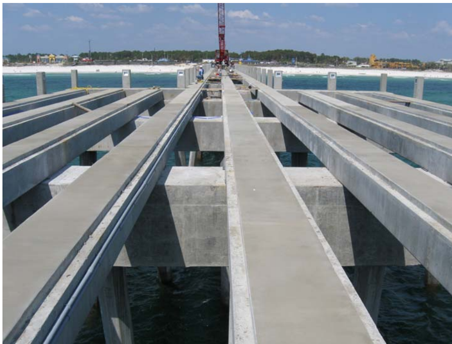
Photo 54. Terminal platform of M.B. Miller Pier prior to deck placement.
