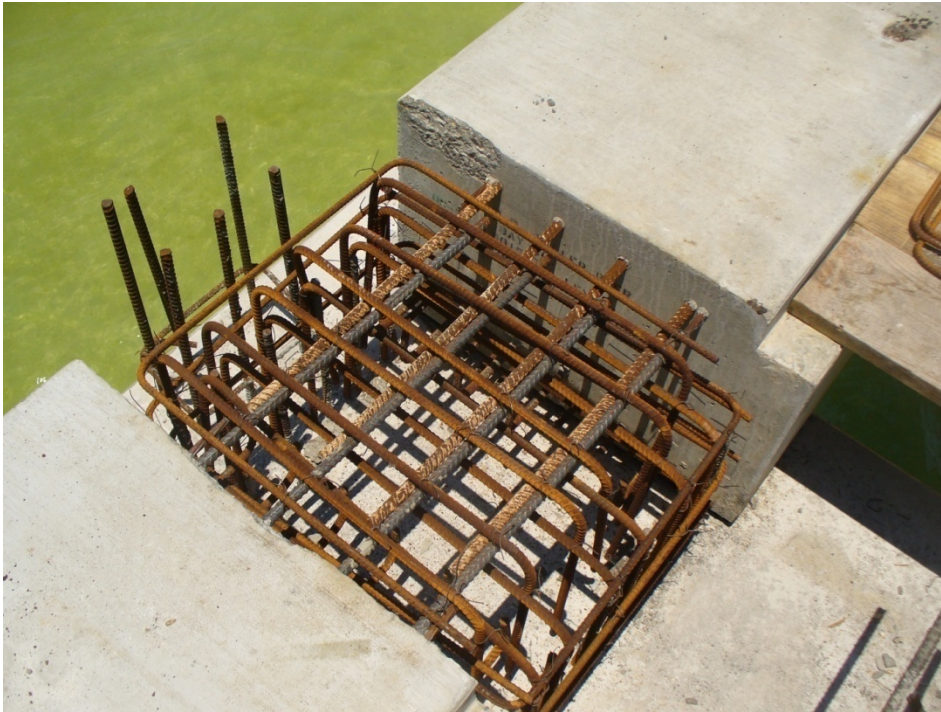
Photo 21. Steel reinforcement on M.B. Miller Pier under construction
