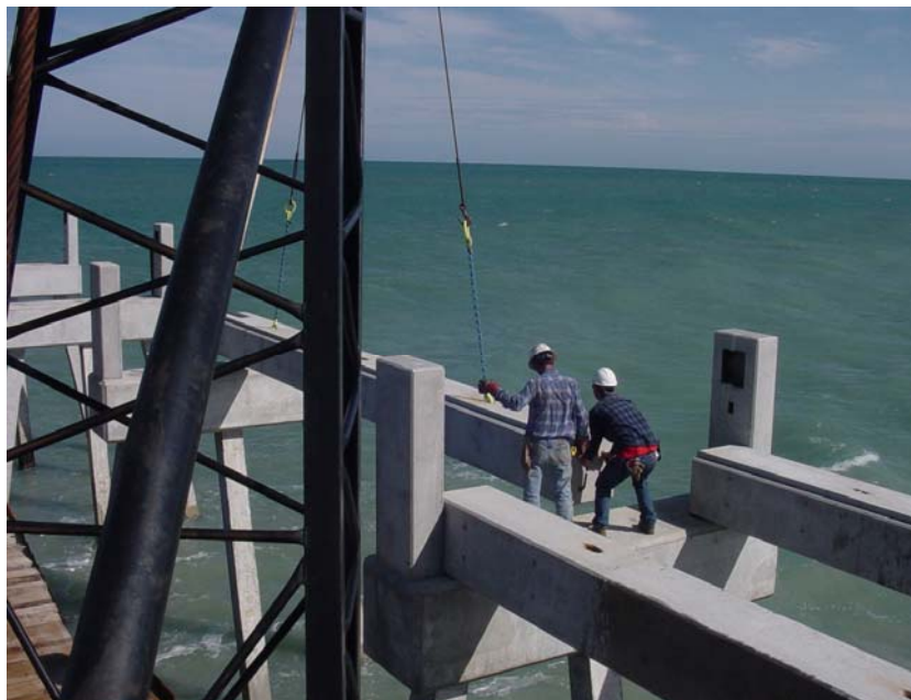
Photo 41. Beam placed on pile caps [Bridge Design Associates, Inc.]
