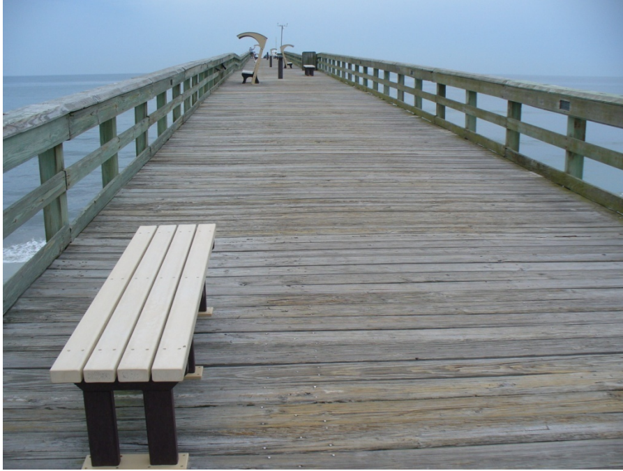
Photo 30. Wood deck planks on concrete St. Augustine Beach Fishing Pier
