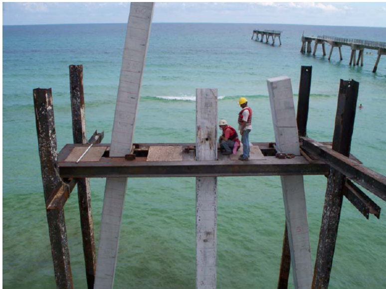
Photo 46. Pile placement template, Navarre Beach Pier [PBS&J]
