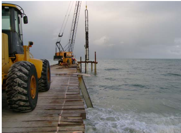
Photo 37. Sea Quay Pier [Bridge Design Associates, Inc.]
