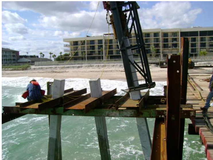
Photo 39. Pile placement template [Bridge Design Associates, Inc.]
