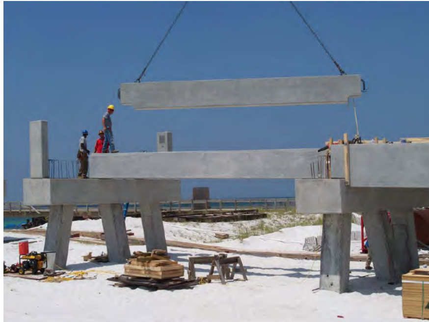
Photo 51. Notched exterior beam placed adjacent interior beam [PBS&J]
