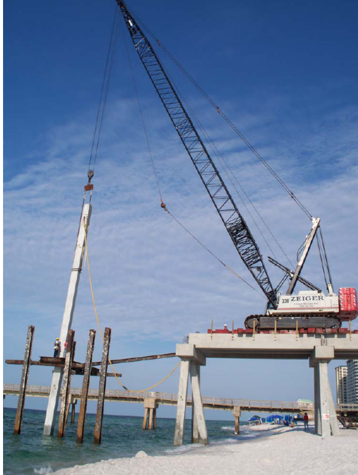
Photo 45. Pile placement by hydraulic jetting, Navarre Beach Pier [PBS&J]
