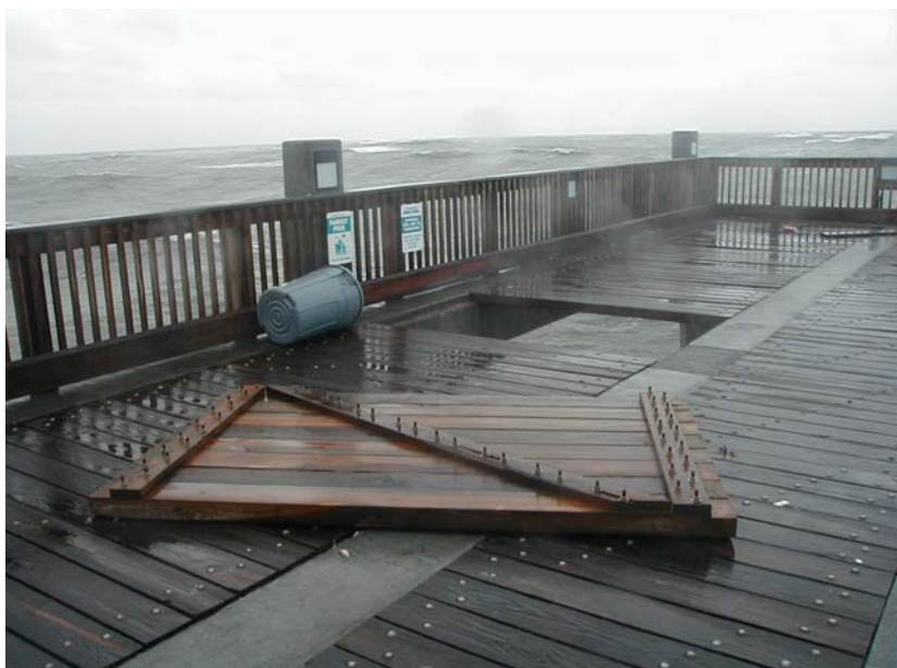
Photo 27. Breakaway pier deck section, Pensacola Beach Fishing Pier
