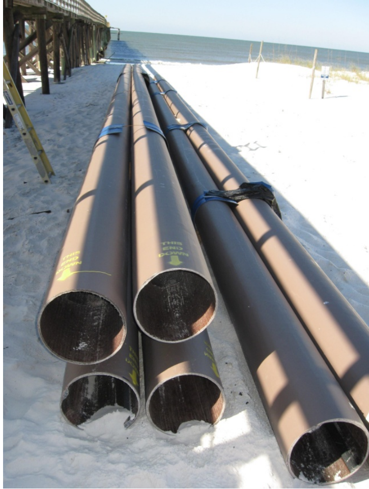
Photo 16. Fiberglass composite piles
