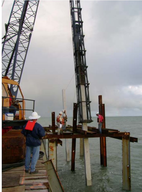
Photo 38. Pile placement with hammer from access trestle [Bridge Design Associates, Inc.]
