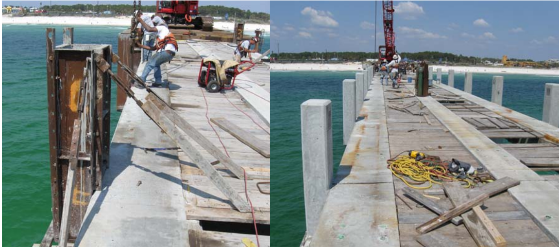
Photo 53. Casting in place the bollards, M.B. Miller Pier
