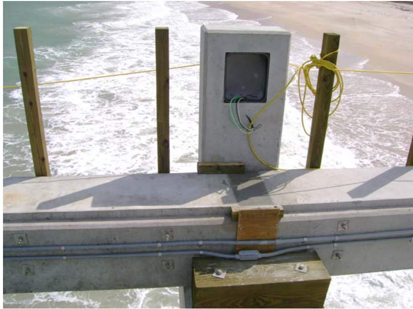
Photo 42. Electrical lines and railing posts [Bridge Design Associates, Inc.]
