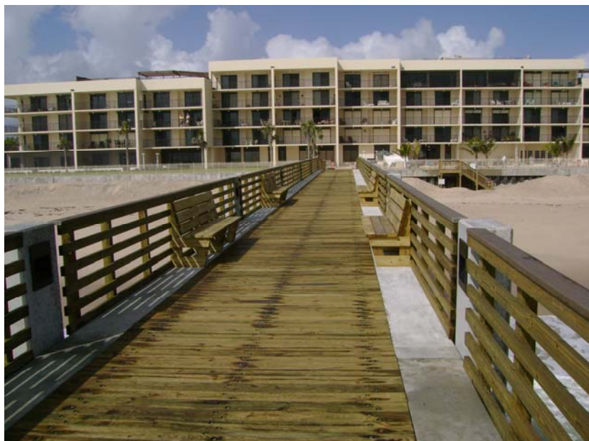
Photo 43. Wood deck and side rails [Bridge Design Associates, Inc.]
