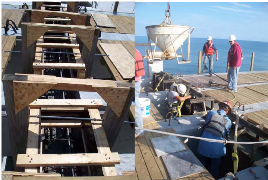
Photo 52. Diaphragm form, left, and casting in place the diaphragm, right [PBS&J]
