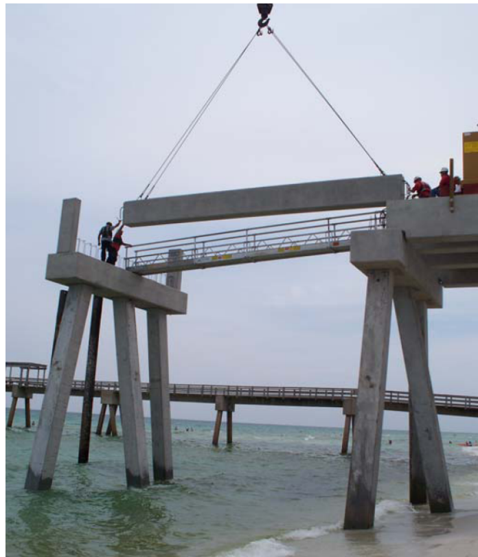
Photo 48. Beam placement by pier mounted crane [PBS&J]
