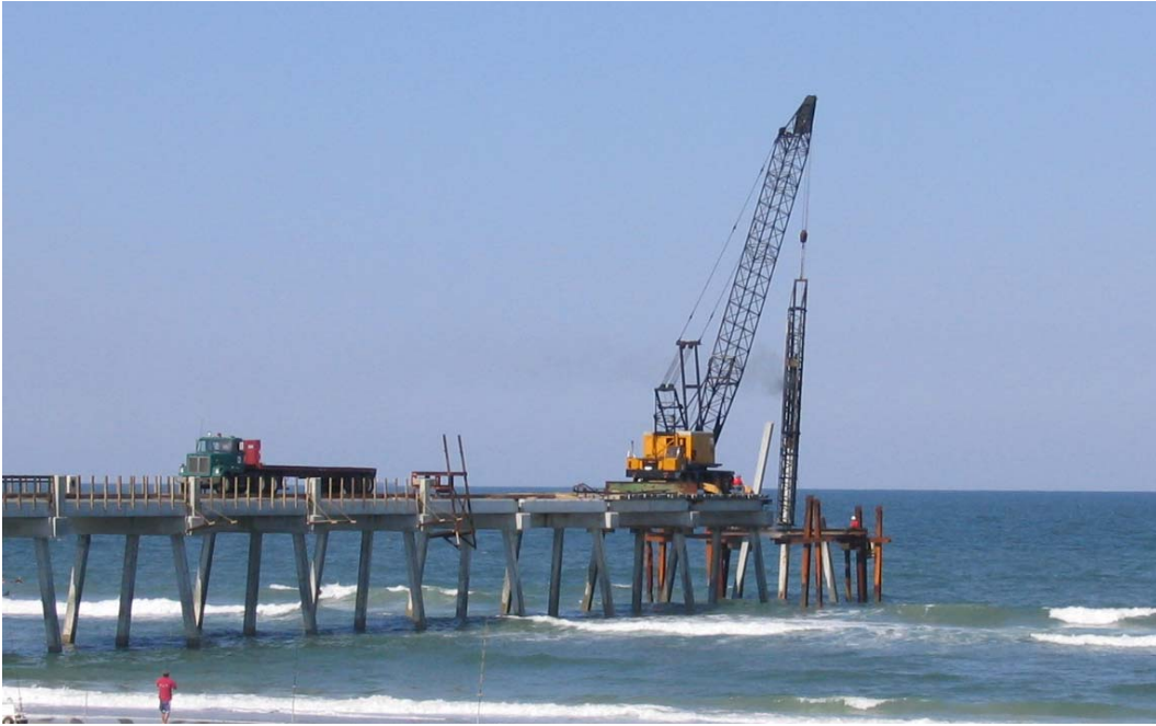
Photo 17. Construction crane and vehicle, Jacksonville Beach Pier [Photo from PBS&J]
