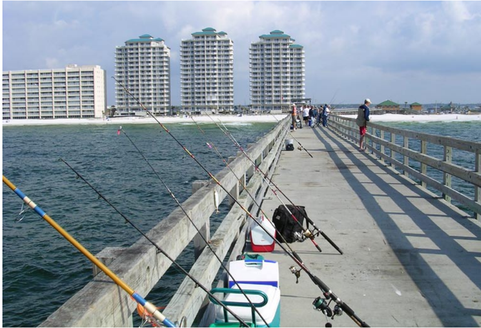
Photo 6. Solid concrete deck, Navarre Pier (1974-2004)
