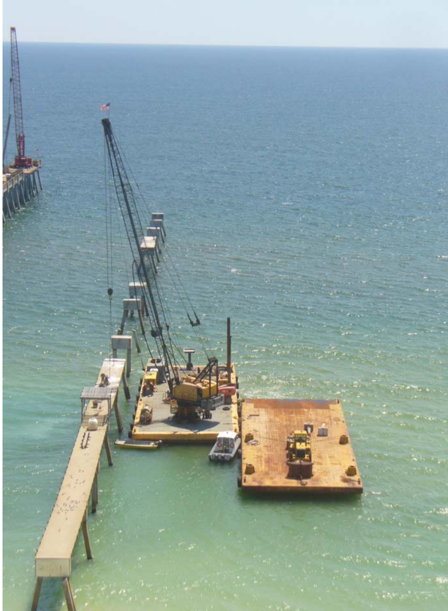
Photo 35. Demolition of old Navarre Pier by barge mounted crane
