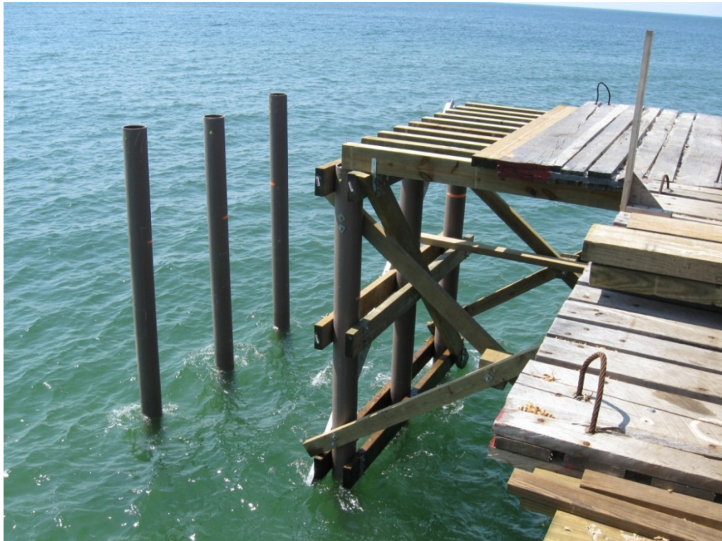
Photo 15. Mexico Beach Pier extension with T-section under construction using fiberglass piles
