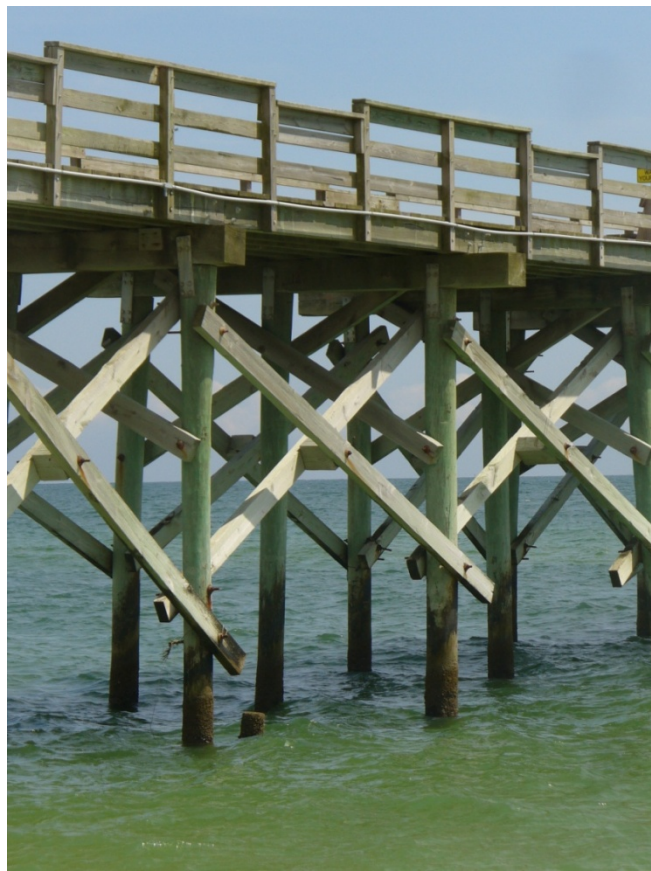
Photo 23. Timber pile and frame
