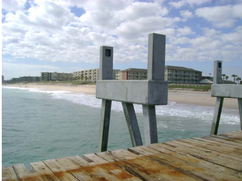
Photo 40. Pile cap with bollards [Bridge Design Associates, Inc.]
