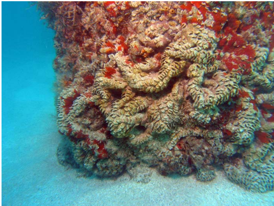
Photo 59. Sabellariid worm rock on pile, Sunny Isles Pier [BBCS Photo Files]
