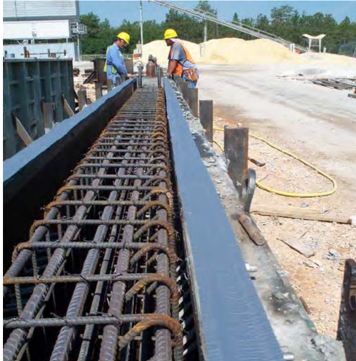
Photo 49. Forming a precast concrete beam off-site [PBS&J]
