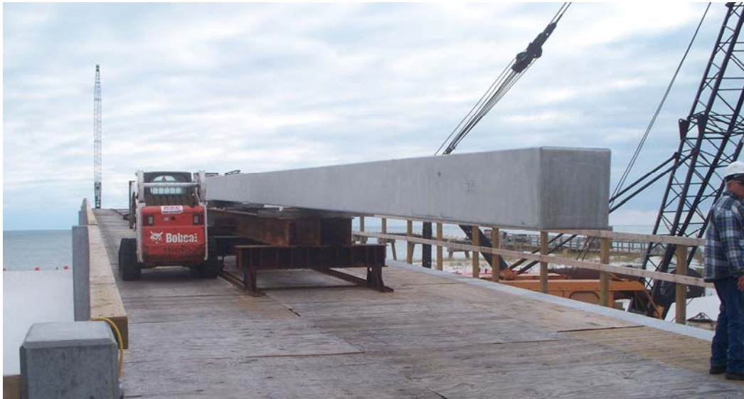
Photo 50. Trolley of steel casters and rails transporting precast piles [PBS&J]
