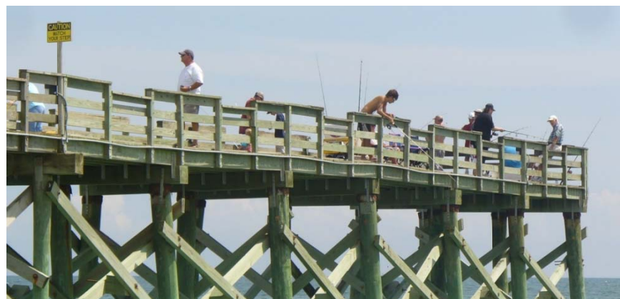
Photo 33. Wheelchair accessible rail segments, Mexico Beach Pier
