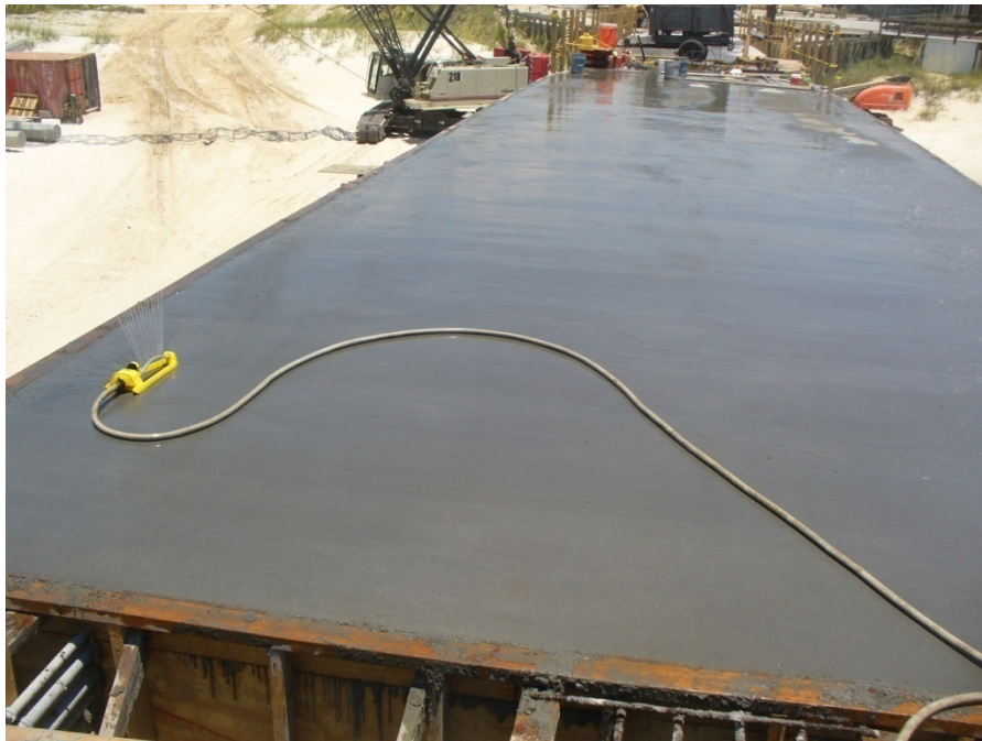
Photo 20. New concrete work on M.B. Miller Pier under construction
