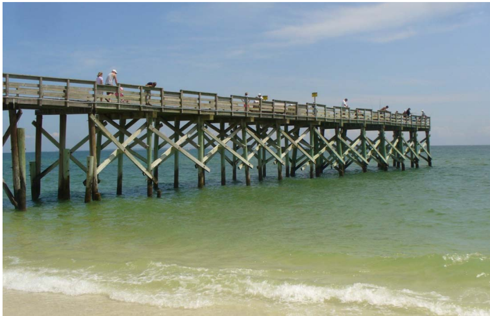
Photo 14. Timber Mexico Beach Pier prior to 2010 extension
