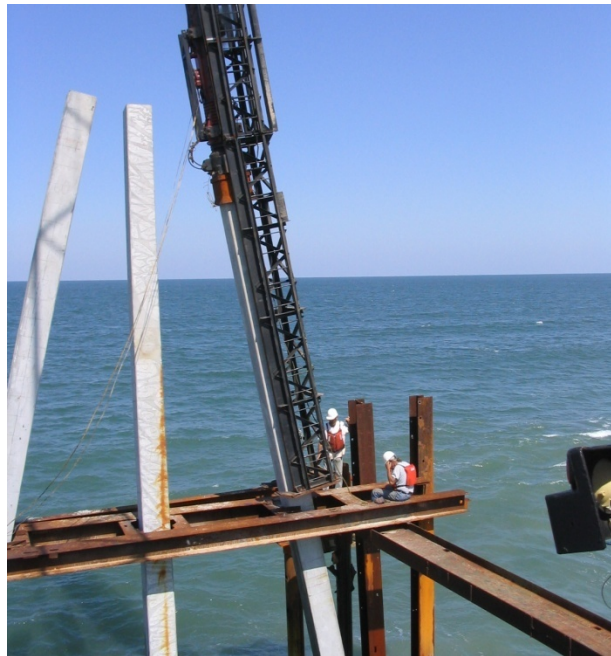
Photo 11. Installation of battered piles.
